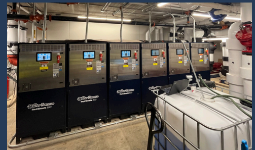
WaterFurnace TruClimate 500 6-Pipe Geothermal Chillers
